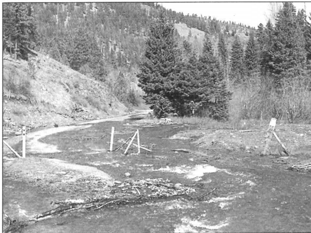
A road under water.
