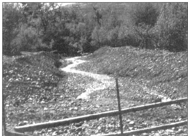
Levees on a heavily used stream.
