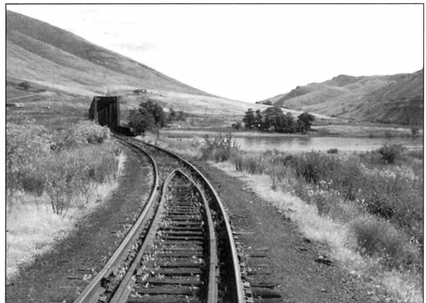
This railroad bed cuts the river off from its floodplain and prevents the formation of marshy areas or backwaters that would absorb some of the force of flooding.
