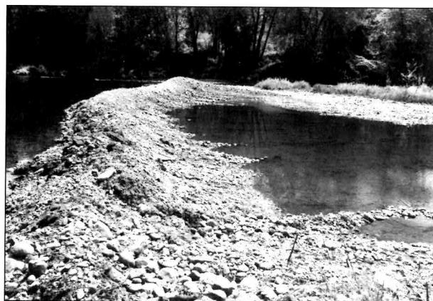
Pushup dams that are constructed yearly for irrigation disturb the stream channel and often block fish passage.
