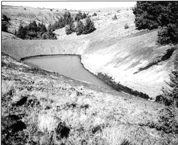
Sediment basin in uplands of Buck Hollow Creek watershed.
