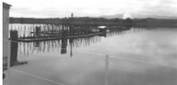
New CEDC Fishery Net Pen facility at East Tongue Point (MERTS Maritime dock). Notice the 21 new steel pilings looking East towards Nicolai Mt. with space available for more pens.
