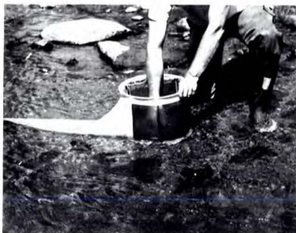
Photo by Dr. Brusven, U of I Plate 5.3 Bottom sampling device used to measure standing crop.
