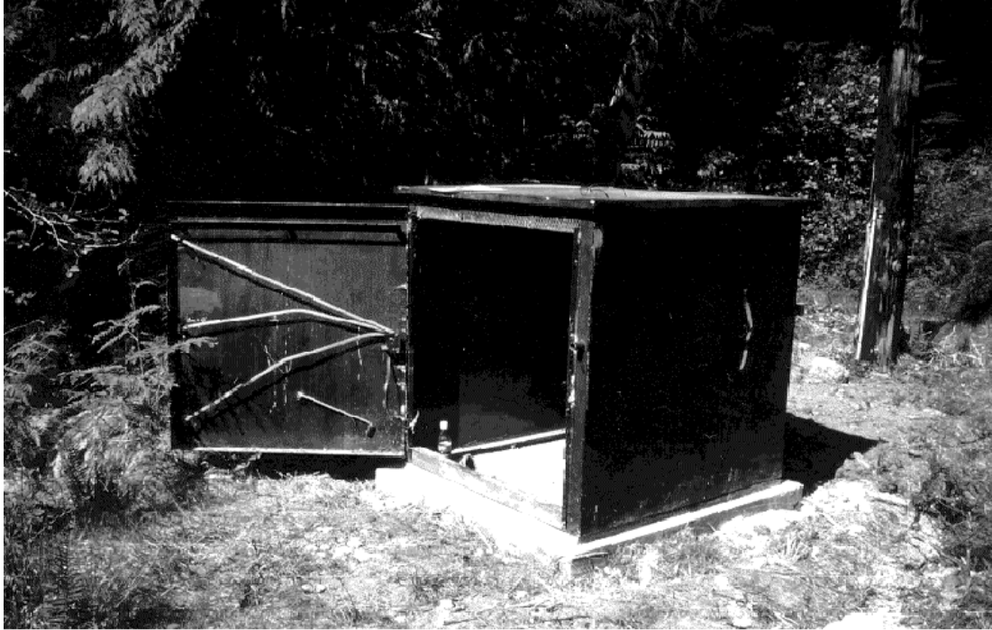
Figure 7. Hydrometric shed constructed on cement pad - Gray Creek pilot monitoring station.
