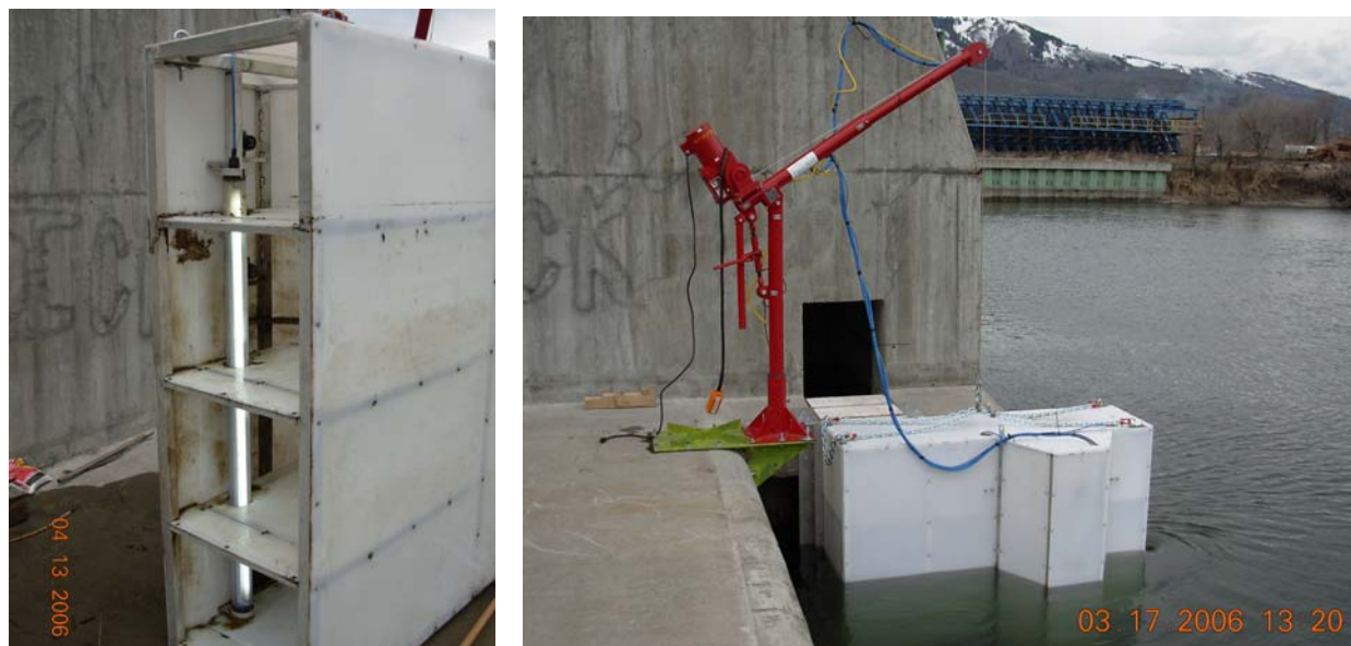
Figure 4. Photographs of Zosel Dam east bank video chute array prior to (left) and during deployment.
