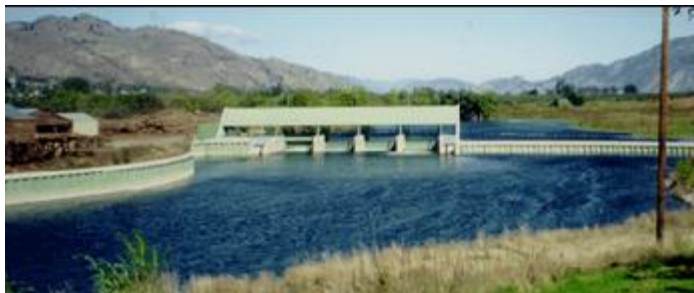
Figure 2. Photograph of Zosel Dam from the tailrace looking upstream.
