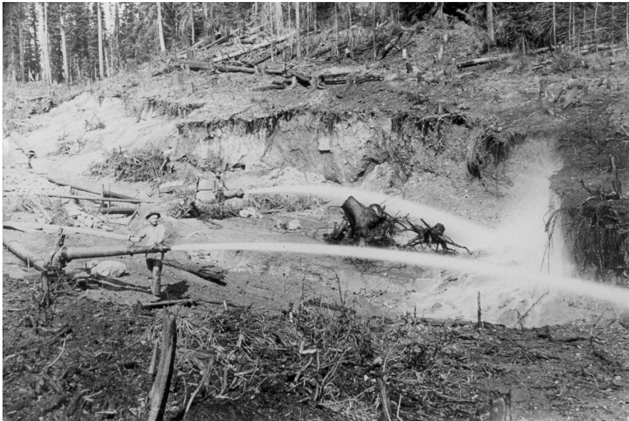
Figure 29 Hydrologic mining on Leggett Creek in the South Fork Clearwater drainage (photo courtesy of Don Morrow)
