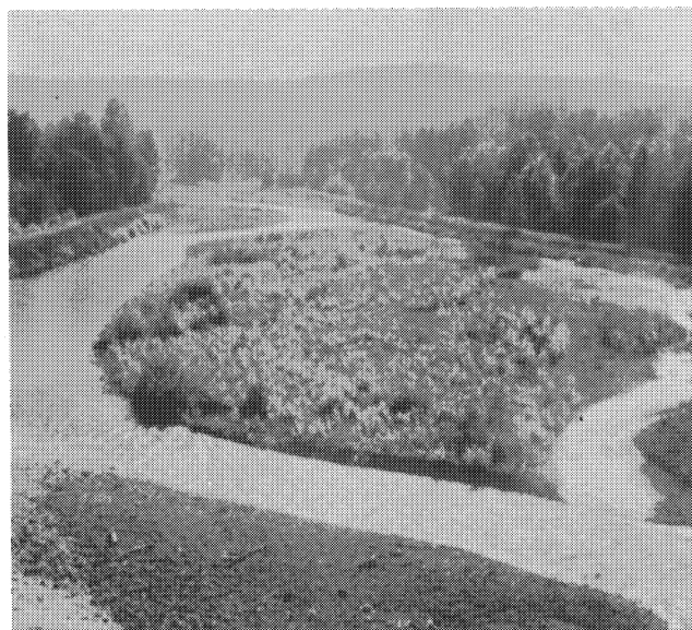
PHOTO 07-21. Set back levees on lower Tolt River allows the river to meander.
