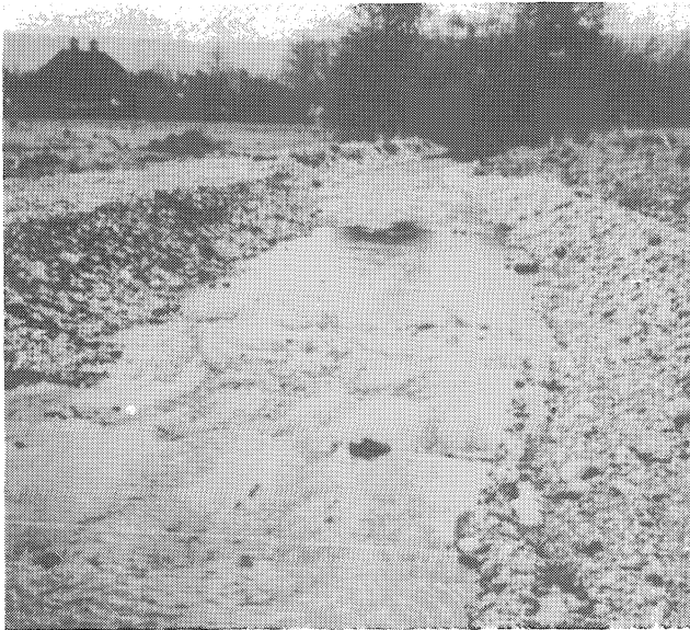
PHOTO 07-13. Channelization can reduce or eliminate fish production. (Griffin Creek)
