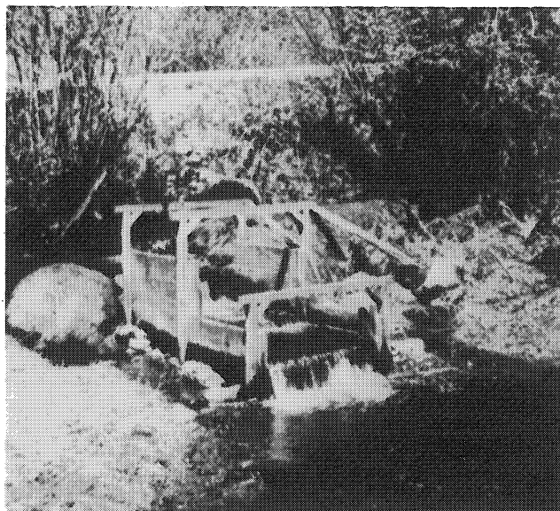
PHOTO 07-20. A two-step fishway through a road culvert on upper Harris Creek.
