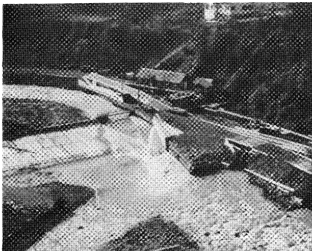
PHOTO 10-13. White River diversion dam.
