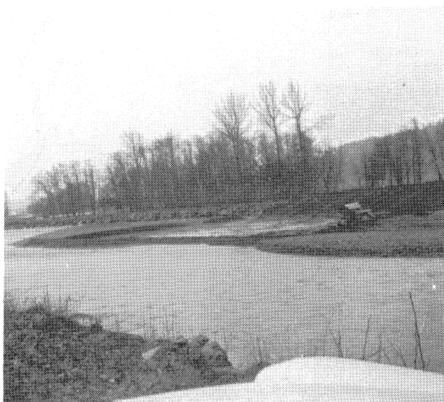
PHOTO 10-16. Flood control diking operations alter the natural stream habitat.
