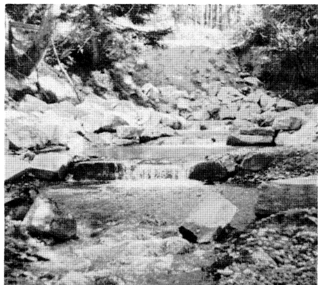
PHOTO 12-5. Streambed controls help fish negotiate poorly designed culverts (Leach Creek).
