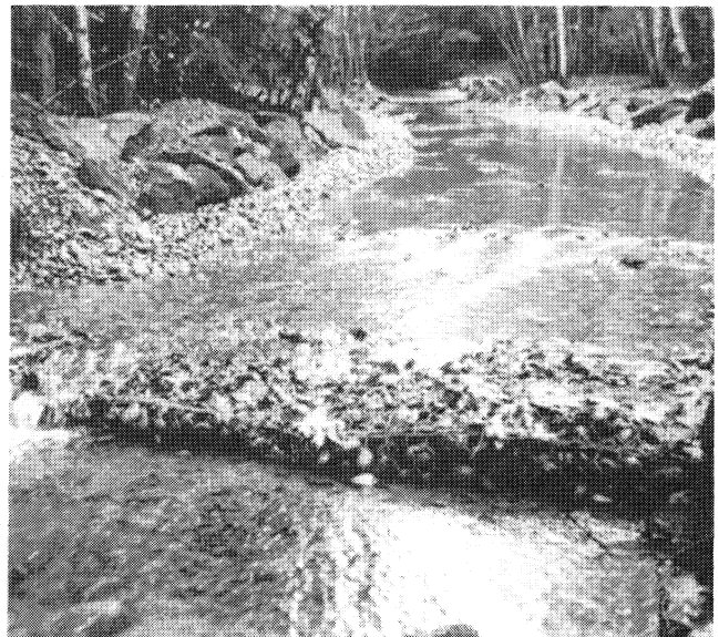
PHOTO 13-10. Streambed stabilization on Swift Creek, tributary to McLane Creek.
