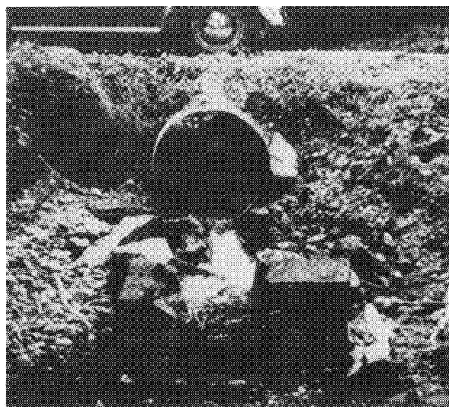
PHOTO 15-5. Improperly placed culverts block migrations to many miles of upstream area (Dewatto Creek tributary).
