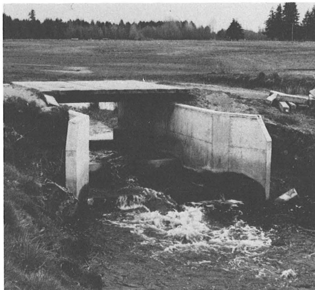
PHOTO 22-21. Fishway on Blooms Ditch diversion dam.
