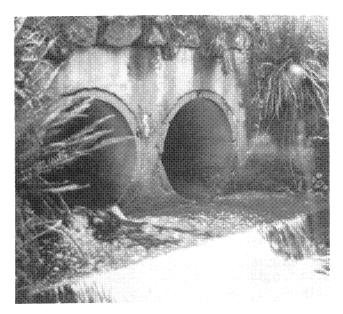
PHOTO 24-7. Road culverts often become migration barriers for adult salmon due to erosion or improper installation (unnamed tributary of Willapa River).
