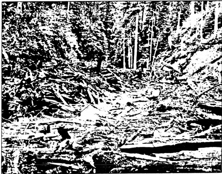
Fig. 2. Log and debris jam removal on West Fork Tilton River. Jam was total block to upstream migrant salmon.
