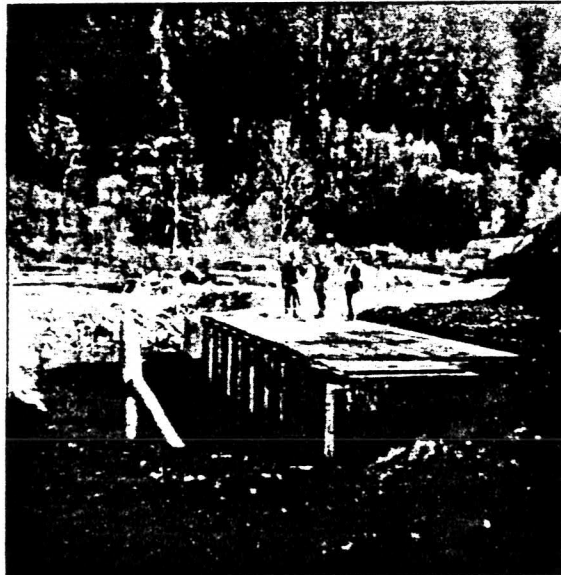
Fig. 6. Toutle Hatchery water supply intake on Green River.
