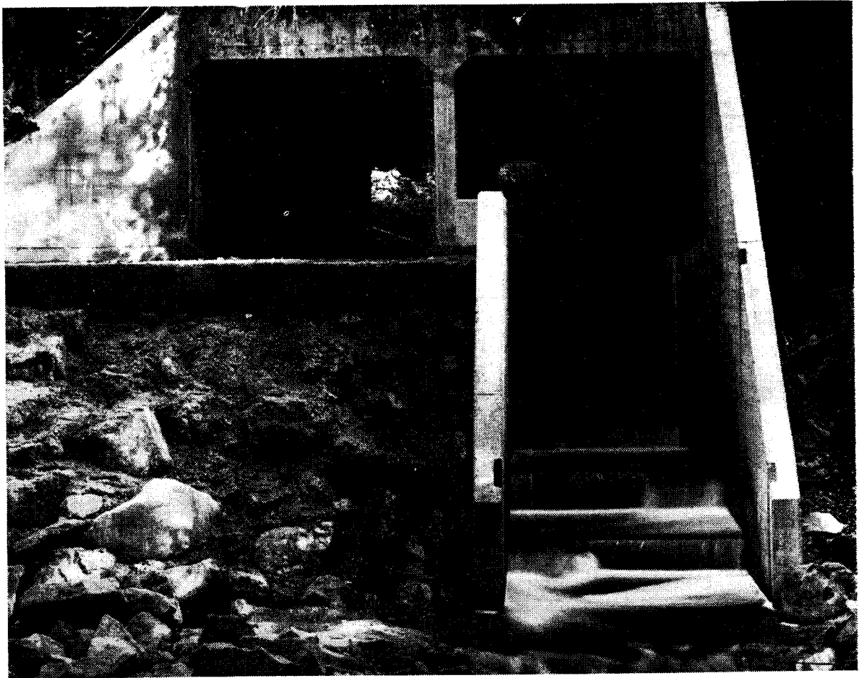
FIGURE 2 —Siebert Creek showing 12-foot erosion of stream bed below culvert and correctional fish ladder installed in one barrel of the culvert. Bagley and Siebert Creeks are on the Olympic peninsula near Port Angeles.
